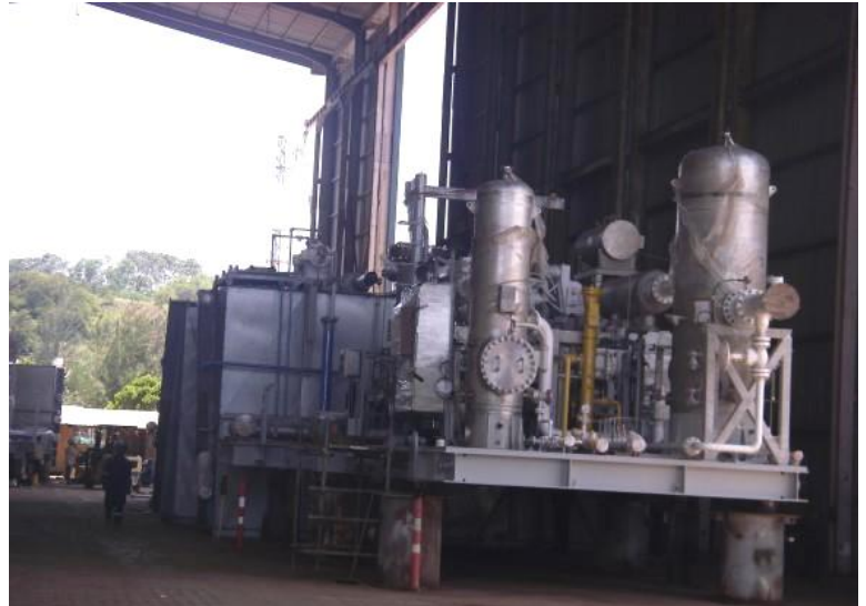
Above: Compressor skids and air-cooler fans were shifted via self-propelled modular trailers (SPMT)
